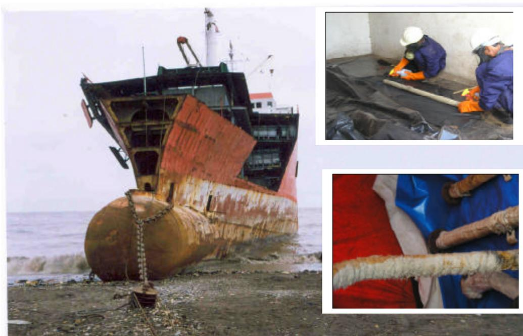
Fig. 1. Source of asbestos exposure during ship breaking
